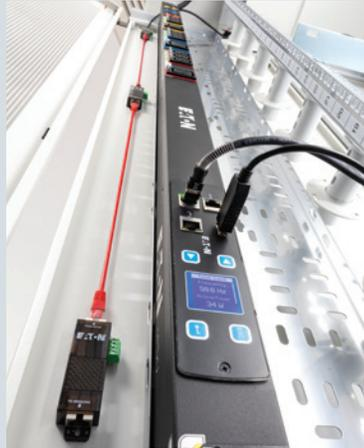
Three daisy-chained environmental monitoring probes with a rack PDU
