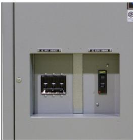
This feature provides thermal-magnetic circuit breakers with higher AIC ratings than the standard. See the tables on Page 10 for medium and high AIC breaker ratings.
